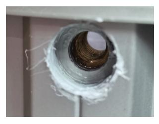
**STEP 2.**Apply Tef-Gel to 4 x M6 Security bolts as shown here
