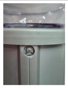
STEP 4 - Remove the black shrink wrap from the light head to activate the system. Your Solar Light Bollard is now installed and operational.
